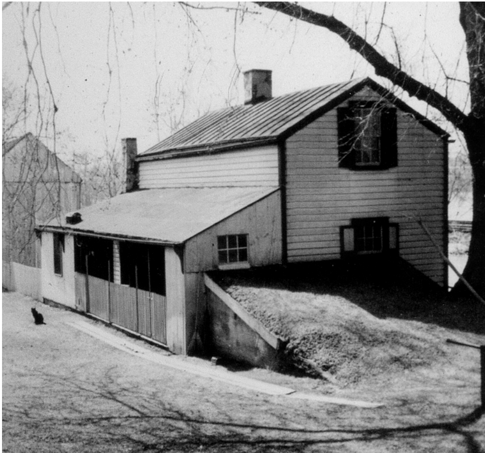
The bridge tenders house at Moore's Station.
