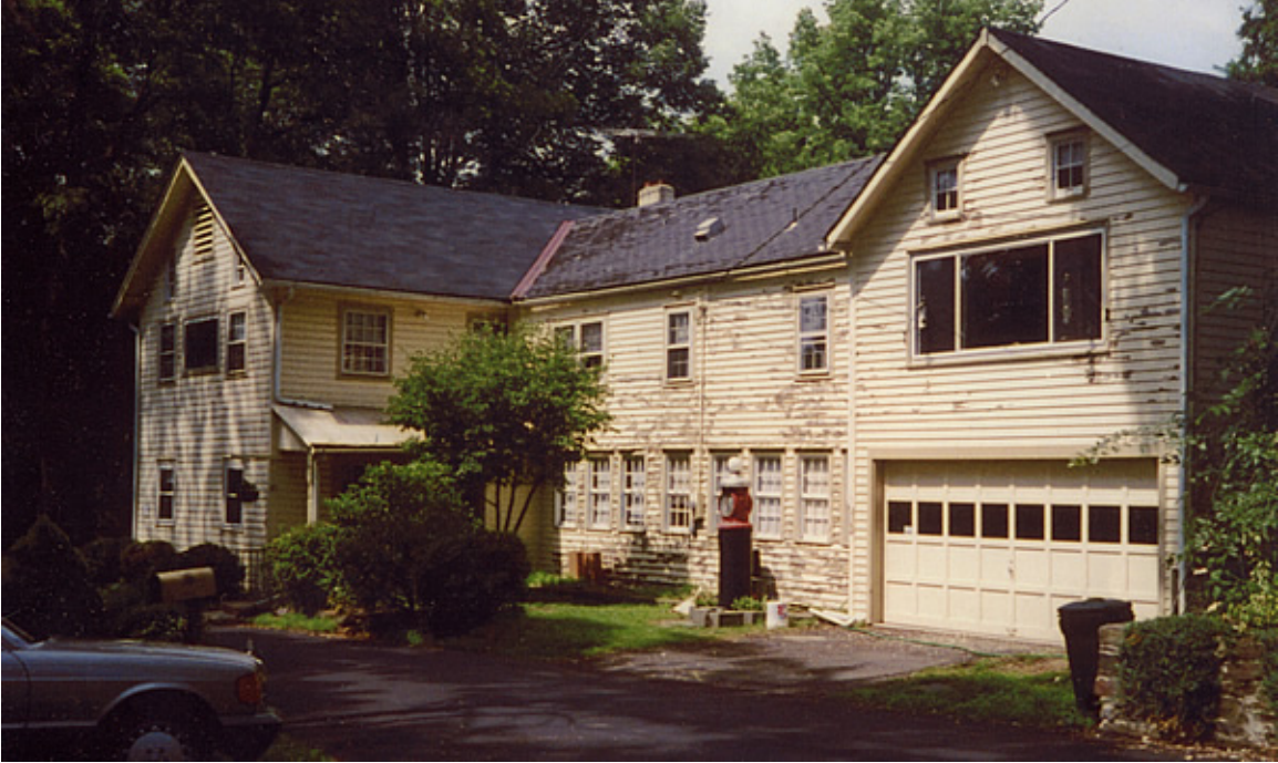
Photo of the canning factory building after its use as the home of the firm of Otto Niederer Sons who manufactured the first successful automatic egg grading machine - the Egg O Matic.
