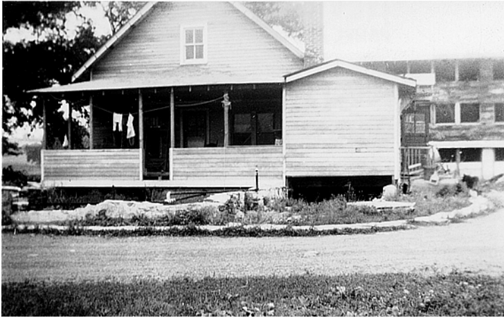
Above: Conversion of the school house into a family home as of 1939. Note the front wall and front porch have been built and the original chimney for the old wood burning cooking stove is in place.
