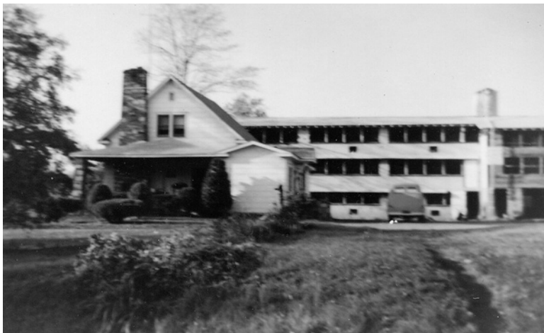
At Right: A 1943 photo showing that the wood stove chimney has been removed and the living room stone fireplace and chimney have been built.
